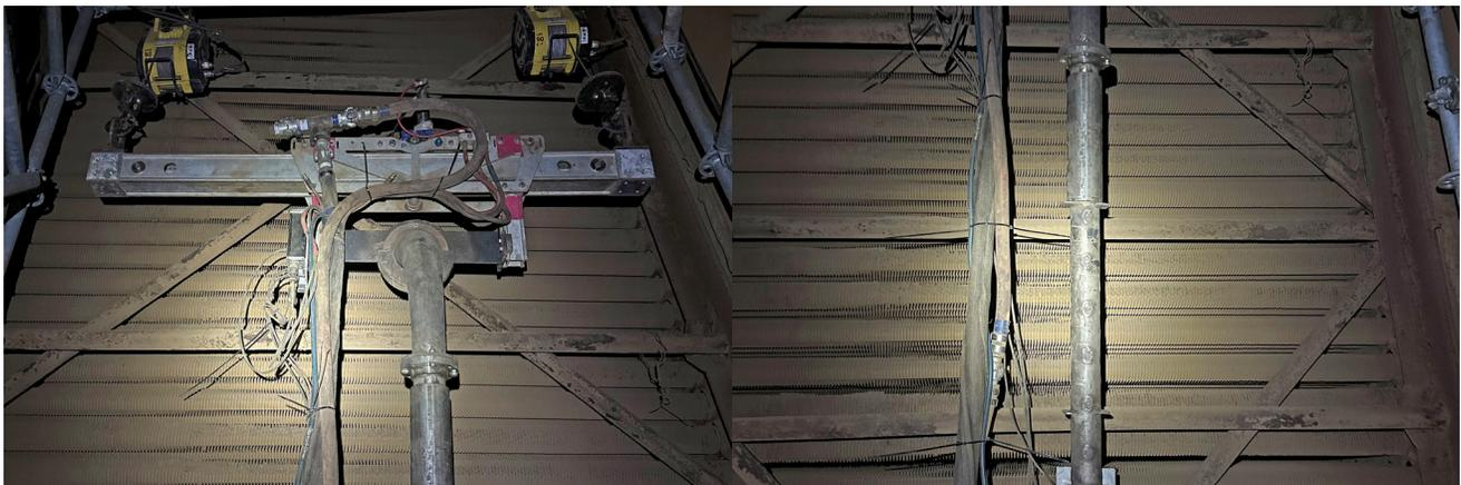
Pictures above provide examples of the condition inside the incinerator prior to the cleaning.
